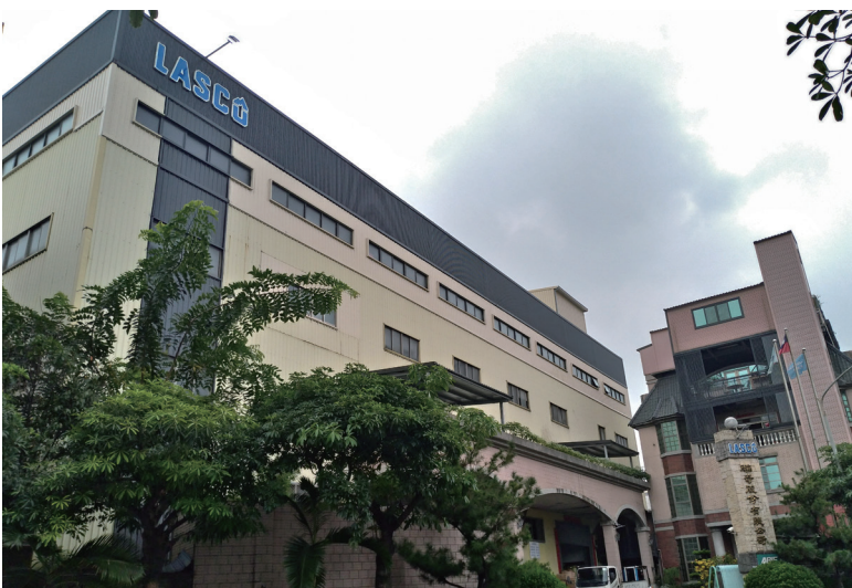
▲ Lunge has expanded its Taichung plant by 1,100m 2 .
